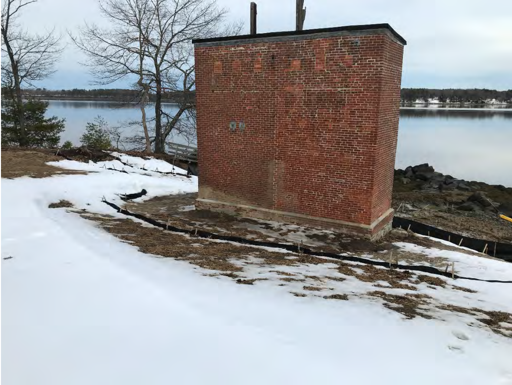
Fig 1: Slope leading down to cable house and salt marsh restoration at the Eversource property/west side of the bay. Viewing northeast. (02-24-21)
