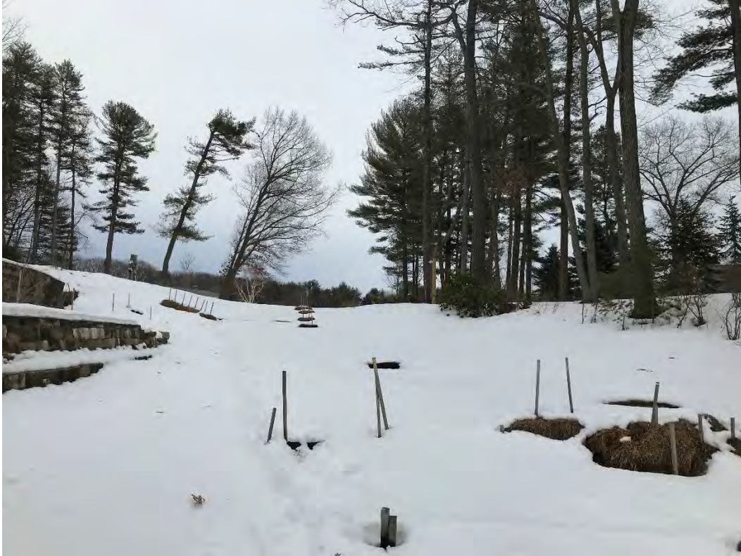
Fig 9: Slope above the manhole at Gundalow Landing/east side of the bay. Viewing east. (02-24-21)
