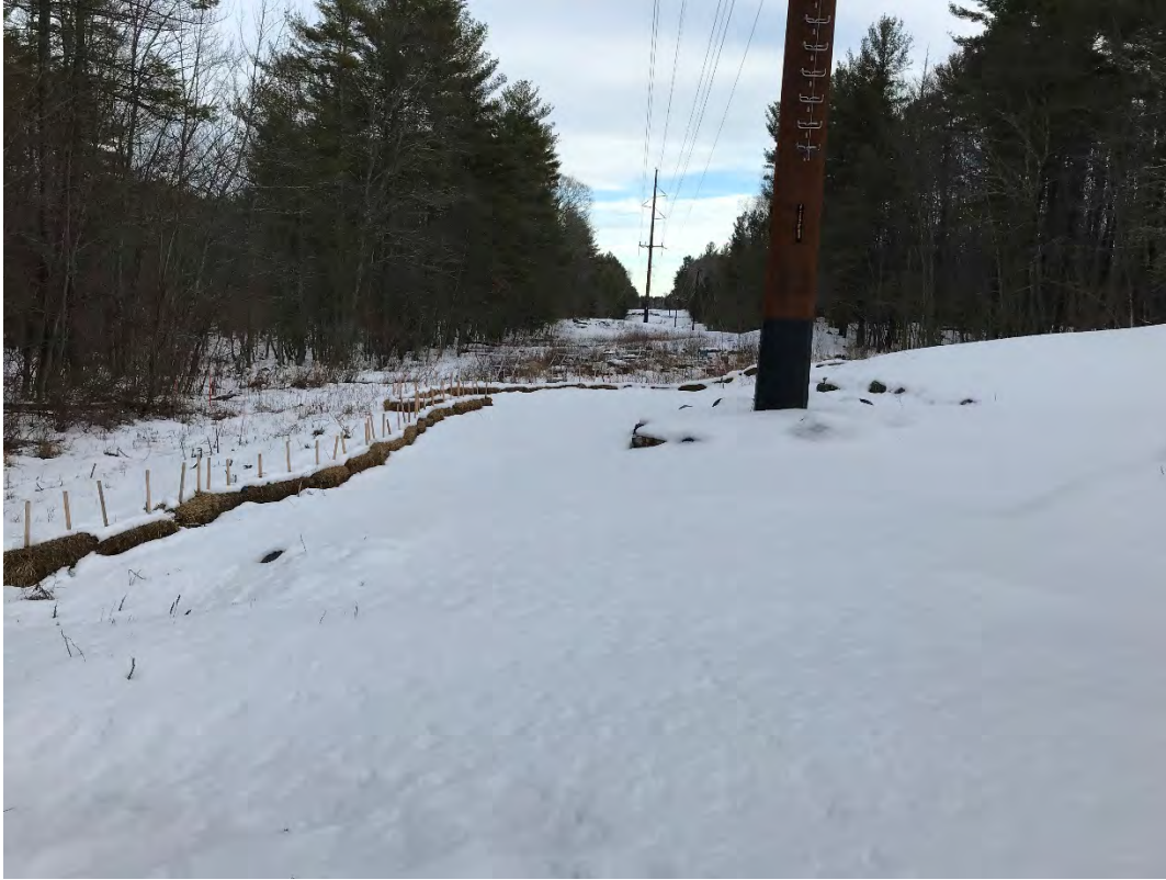
Fig 5: Str. 89 work area. Viewing southeast. (02-24-21)
