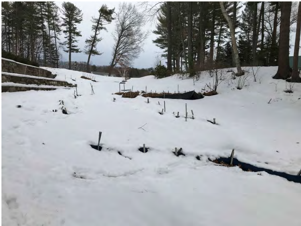
Fig 10: Slope below the manhole at Gundalow Landing/east side of the bay. Viewing east. (02-24-21)
